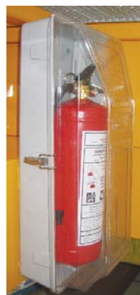
Fire extinguisher in locker
