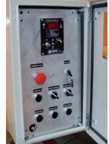
Electrical control of valves and remote control as option
